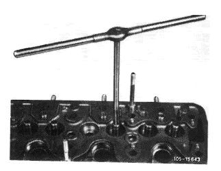
9 Check inside diameter of valve guide with plug gauge.
